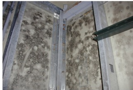
Pressure release valve stuck open with rust
