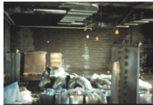
Expansion joint leak
