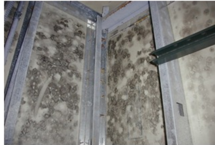
Pressure release valve stuck open with rust 59
