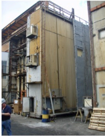
Thermal Testing by Cooling
