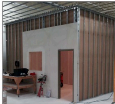
MOCK UP ROOM CREATED TO TEST WALL PENETRATIONS WITH A BLOWER DOOR
