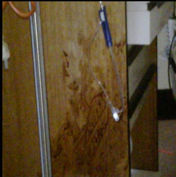
Inadequately cleaned surface in patient room. Major teaching hospital, Sydney. 2008. Taken by patient's family and supplied to Infection Control Plus. 37
