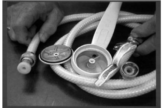
Bio-film on the inside of plumbing fixtures
