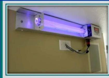
\* A high photon energy lamp that is safe for people. It falls below the FDA threshold limit value (THV) for human exposure, it's used to disinfect air and surfaces from
